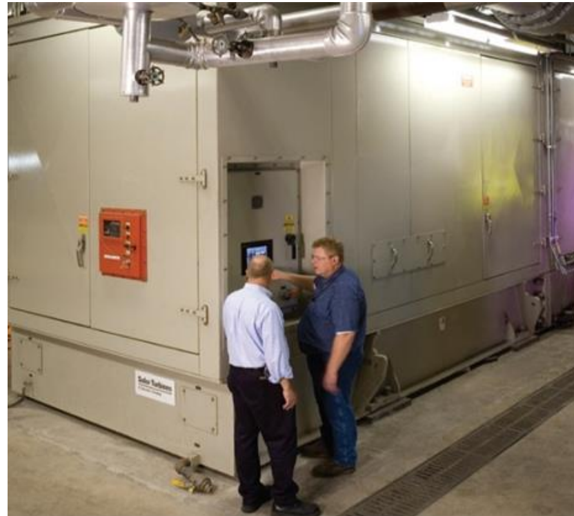
15 MW gas turbine generator set at Michigan State Univ., Solar Turbines Inc.
