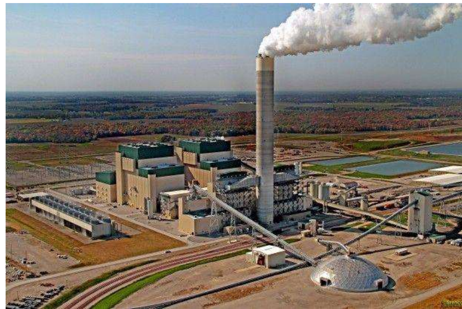
Prairie State Energy Power Plant
