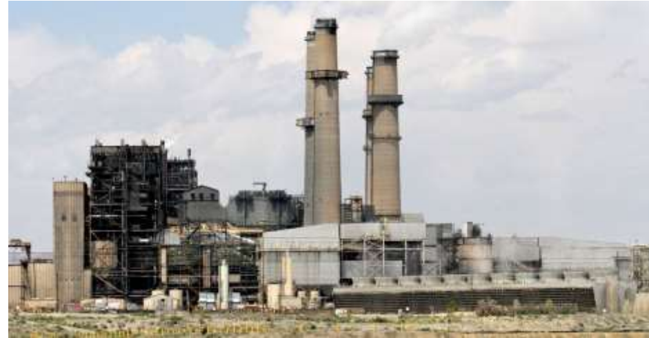
San Juan Generating Station
