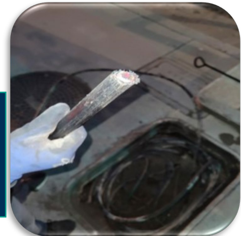
Underground vault and two risers accessed; cuts made to 3 fiber lines. Santa Clarita, CA May 2024
