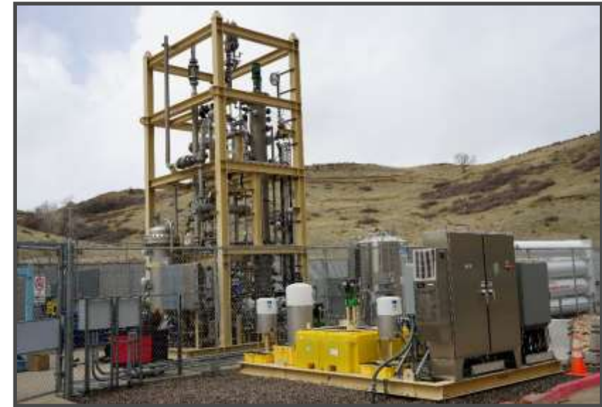
700 Liter Vertical Stirred Biomethanation reactor at NREL
