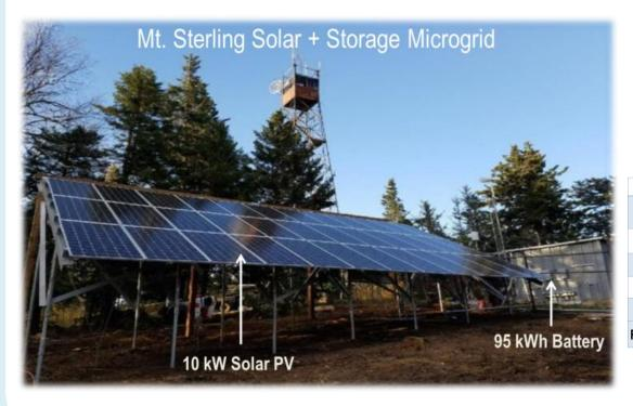
Utility-owned and -operated microgrid that serves a remote customer off-grid through 10 kW solar PV + 95 kWh battery
