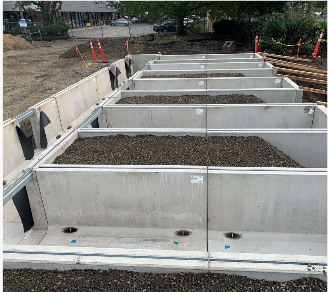
Pre-cast concrete trenches during construction
