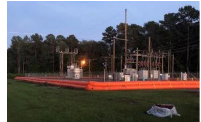
Grifton Station with Tiger Dam Before Hurricane Florence 2018
