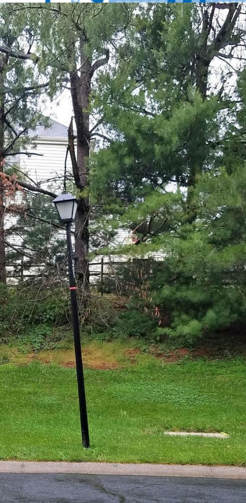
14' to 16' Colonial Streetlight Replaced with 19' to 20' side mounted or ground cabinet
