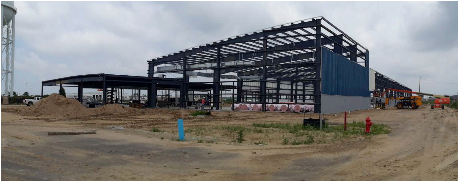
Construction of Sediver's Manufacturing Facility in West Memphis, AR
