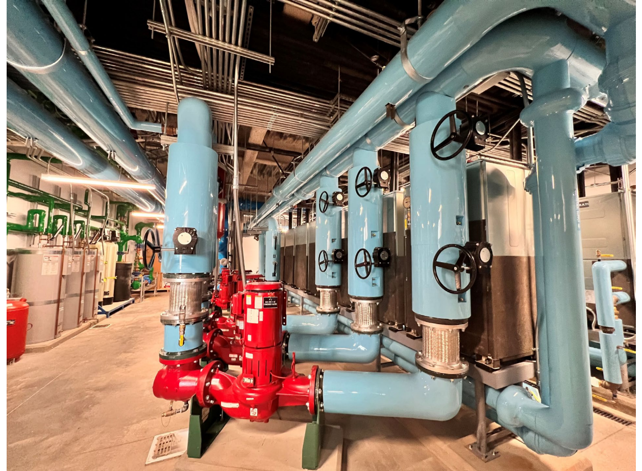
Geothermal heating and cooling system at the University of Utah. Photo courtesy University of Utah.
