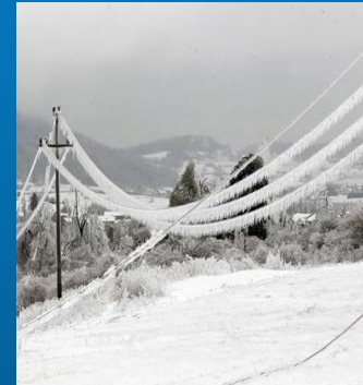
Iced Conductors
