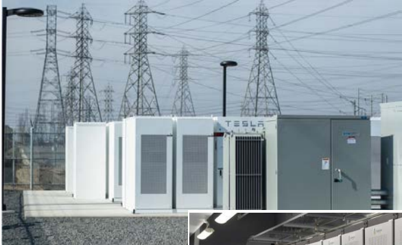
20MW, 4 hours-SCE TESLA, constructed in 88 days
