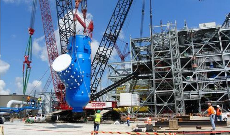
Part of the gasifier – the core of the IGCC process.Gasifiers are assembled section by section
