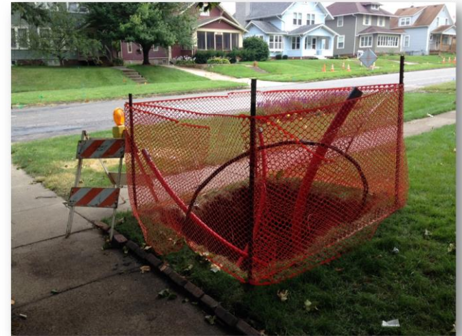
Properly marked and protected pits
