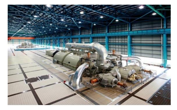
Turbines; Siemens licensed, 1000MW, single shaft, four casings & four exhausts, double backpressures.
