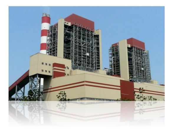
**Boilers**: Alstom licensed, tower type, USC, single reheat, single furnace, corner tangential firing and open arrangement, balanced draft, solid slag disposal, built-in separator, spiral water wall with sliding operation.
