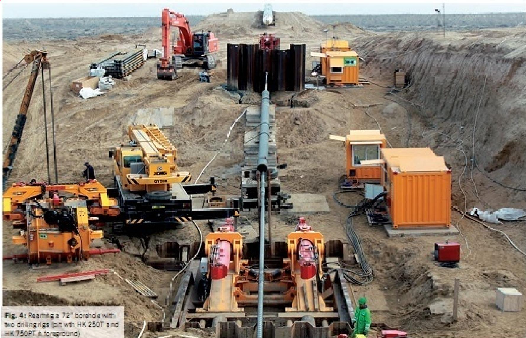
Fig. 4: Reaming a 72" borehole with two drilling rigs (bit with HK 250T and HK 750PT in foreground)
