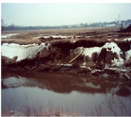
On February 22, 2004, this pipeline broke at a river crossing. 3,000 customers were without gas for two days.
