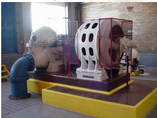
Water Treatment Plant High Service Pump
